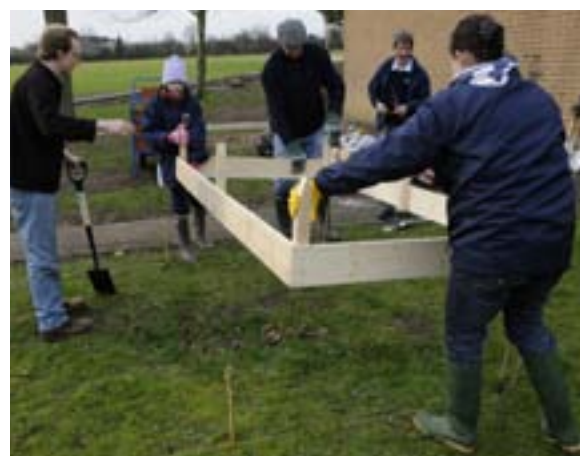
Building a raised bed.
