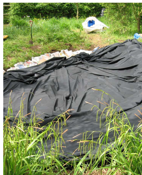
Laying pond liner for new pond.
